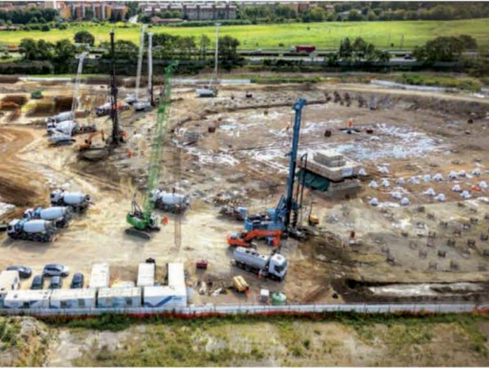
The work involved 883 piles using CFA technology
