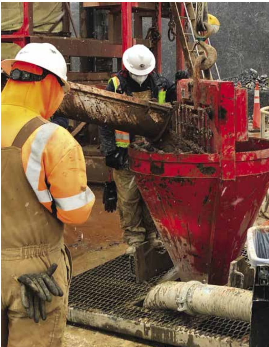
➤ Backfilling of a pile, using tremie concrete Picture: https://twitter.com/BooneRepair/status/1356619037627863045/photo/2
