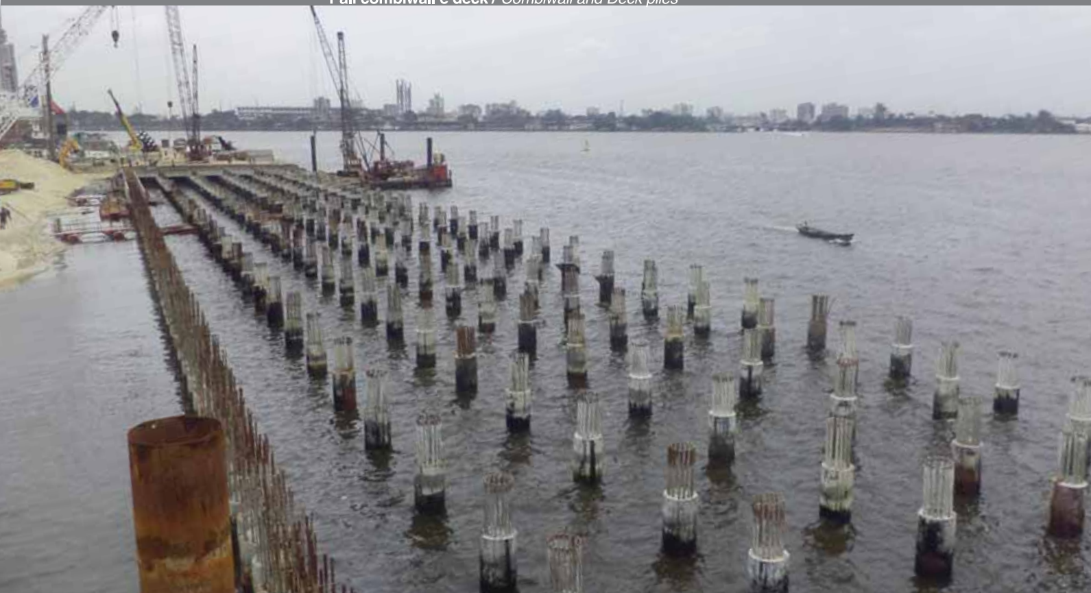
Pali combiwall e deck / Combiwall and Deck piles
