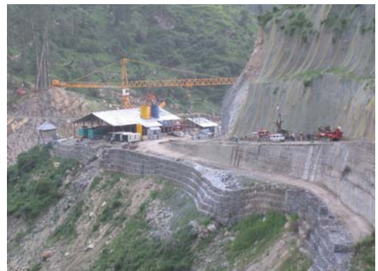
Parbati Hydroelectric Project, Himachal Pradesh, India (2006-2008) – Waterproofing injection for the construction of a cut-off wall in the Paleo riverbed
