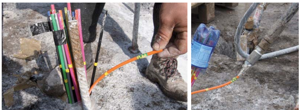
TMG system: grouting through single-valve tubes
