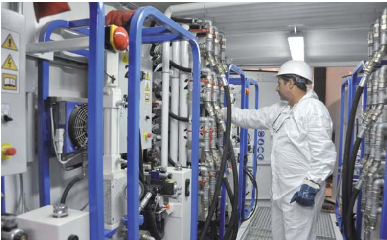
SOILMEC SGJ-8 grouting plant
