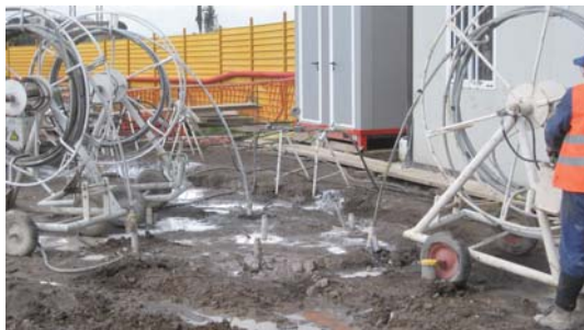
Rome underground: Line C (2010) TAM grouting in loose soil
