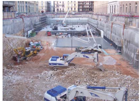
New car park in Piazza Cesare Battisti, Bari (2006/7) – Injection of limestone in Bari to allow for excavation under water table and close to adjacent historical buildings
