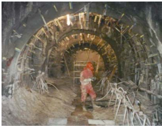
Temporary injection - Milan Underground, Line 3. Waterproofing and consolidation injection.
