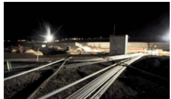
Grout delivery pipes under pressure
